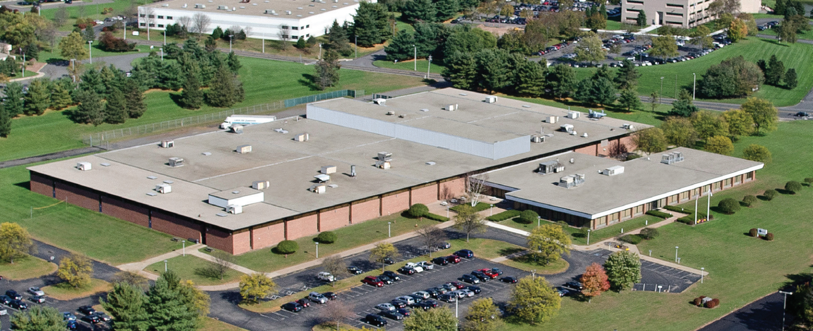
Spencer Corporate Headquarters and Manufacturing Plant, Windsor, CT USA
